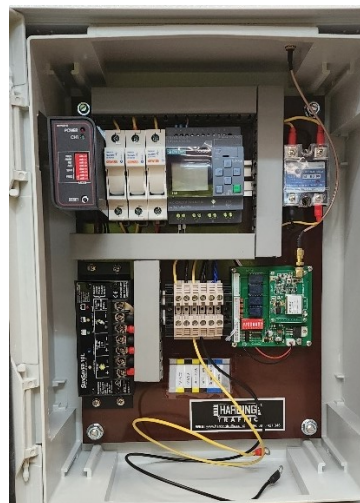
Sign activated via Loop Detector
