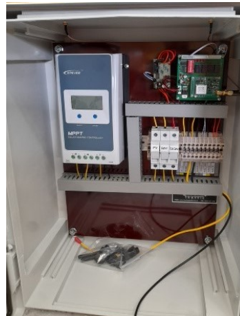
Sign activated via Push Button on Pole
